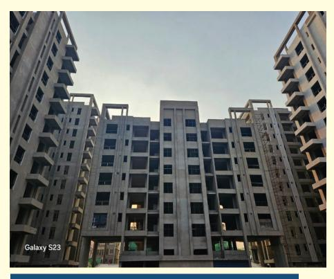
**Tower Tritiya** - External plaster work is completed and window frame fixing work is in progress.
