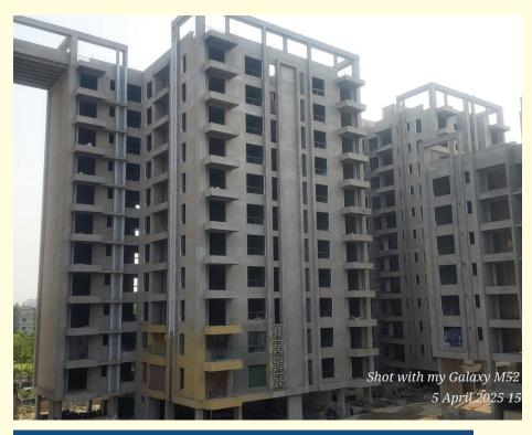
**Tower Chaturthi** - External plastering work is completed & Window Frame fixing work is in progress.
