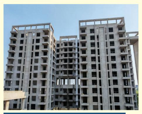
**Tower Panchami** - External plaster work is completed and white wash and shutter fixing work is in progress.
