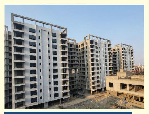
**Tower Prathama** - External plaster work is completed and window shutter fixing and white wash is in progress.
